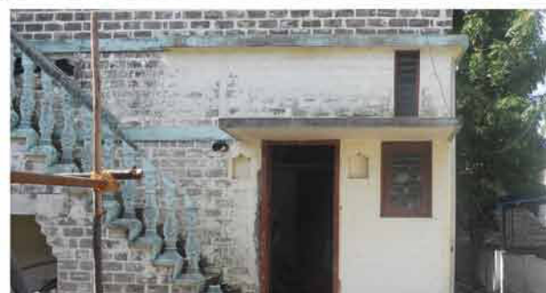
Low-cost housing and sanitation units in tsunami-hit Kodyampalayam, Tamil Nadu, built using fly-ash stabilised blocks
