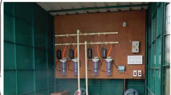
The high throughput ozonator powered by solar energy that is used to disinfect grey water
