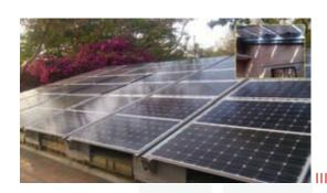
A recently upgraded 9kW, Building Integrated Photovoltaic system (BIPV) facility with an inset of indoor natural lighting (Aaditya G and Mani M. BIPV: A Real-Time Building Performance Study for a Roof-Integrated Facility. International Journal of Sustainable Energy. 2016. 35:1-19).
