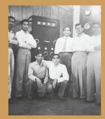
A 1943 photograph of students of the Department of Electrical Technology standing before a 300-watt transmitter that they designed and fabricated for the Royal Air Force, for communication with London during World War II.
