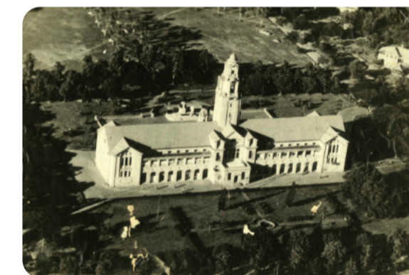
The completed Main Building
