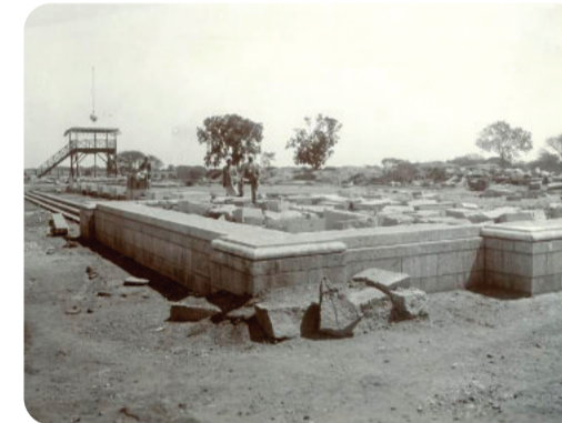
Early stages of construction of the Main Building
