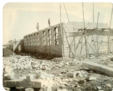
Chemistry lab under construction
