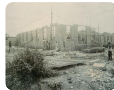
Electrical lab under construction
