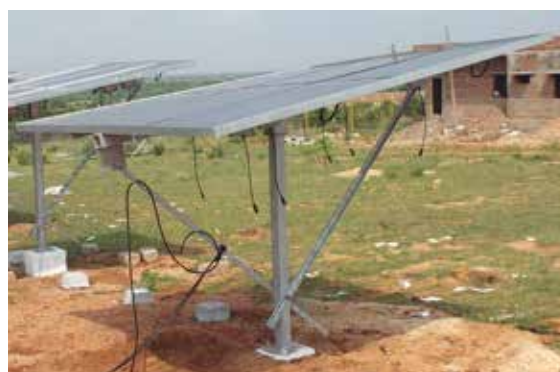
A solar panel pedestal
