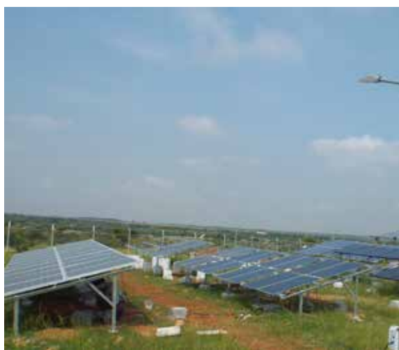
The photovoltaic test-bed at Challakere
