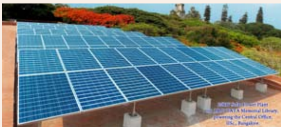
Solar power plant set up on JRD Memorial Library rooftop by Sheela Ramasesha’s group
