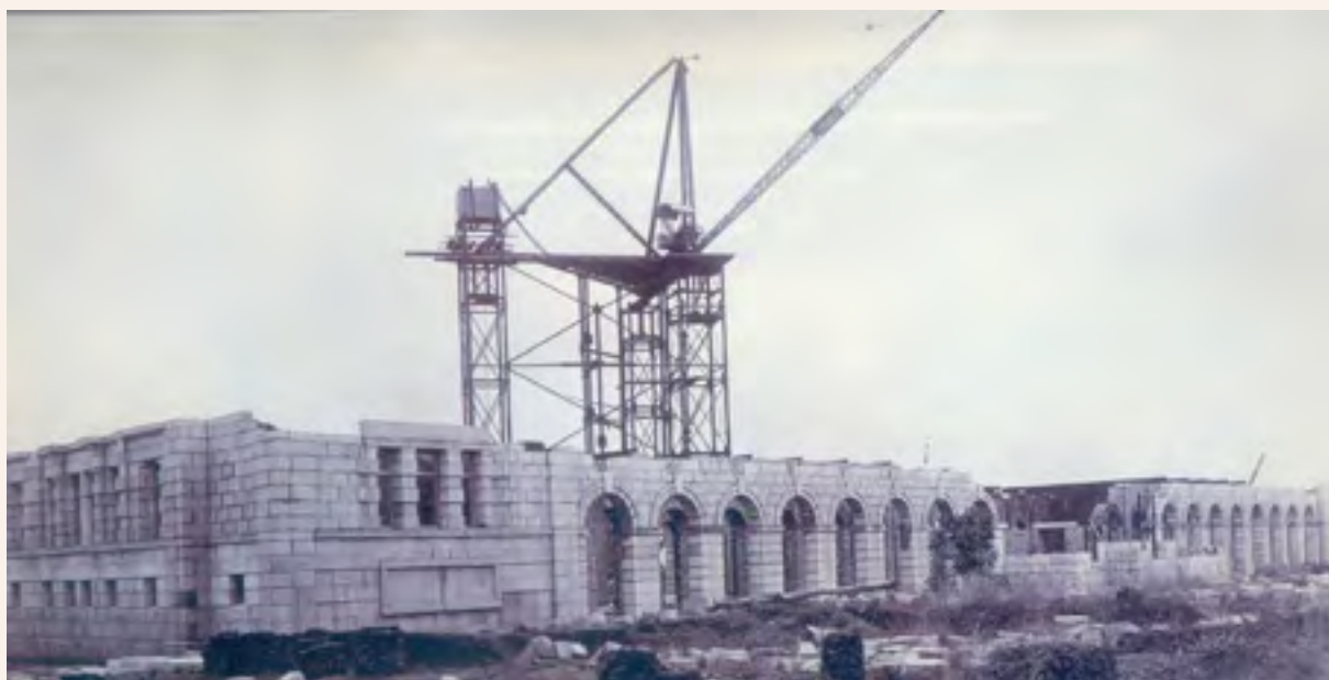
The Main Building under construction
