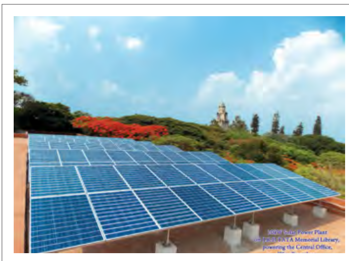
A 20 kW solar power plant on the roof of the JRD Tata Memorial Library to power part of the Central Office at IISc
